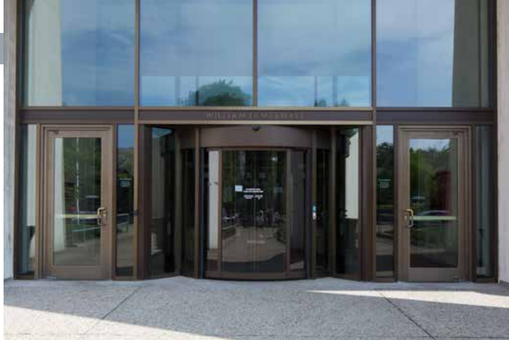
Main entrance to William James Hall features Ellison Bronze doors made from extruded aluminum.
