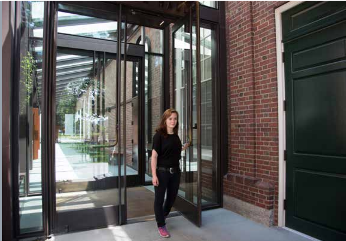
Ellison custom balanced doors grace the reconfigured McKinlock Hall, an undergraduate residential section of Harvard's Leverett House.
