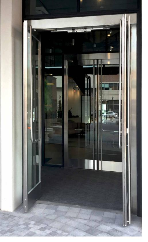
Balanced doors also offer a unique advantage due to their distinctive design that leads to smooth operation. The pivot point, located at two-thirds of the door's width, creates a more balanced fulcrum point for distributing the door's weight, allowing for larger and heavier doors to be opened with ease. This design also results in a reduced door swing area, making them ideal for spaces with a tighter footprint, or municipalities that have strict sidewalk projection codes.
